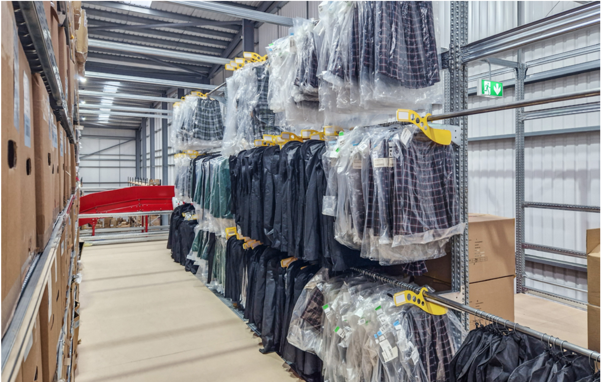
Super 4-5-6 Fashion Multi-Level Warehouse Reference Installation <August 2024>
