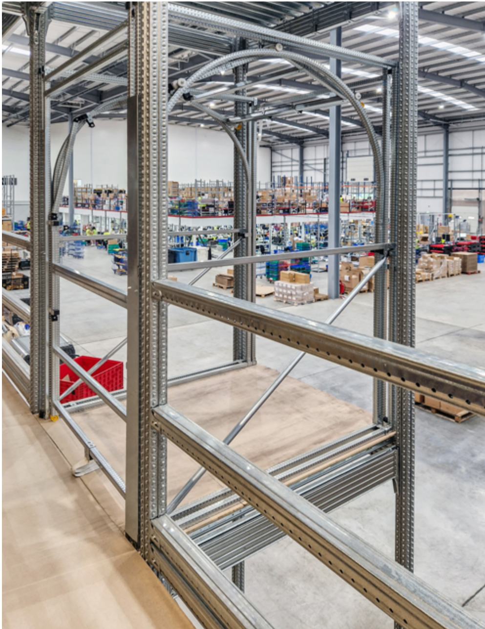
Super 4-5-6 Fashion Multi-Level Warehouse Reference Installation <August 2024>
